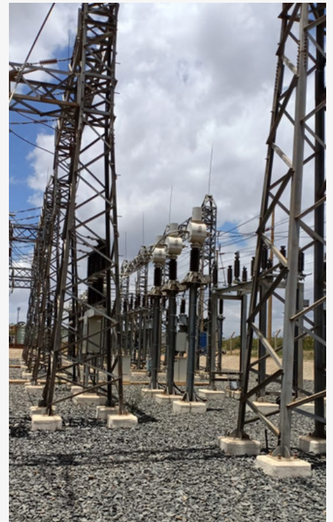
Commissioning of 33KVA Substation at Lamu
