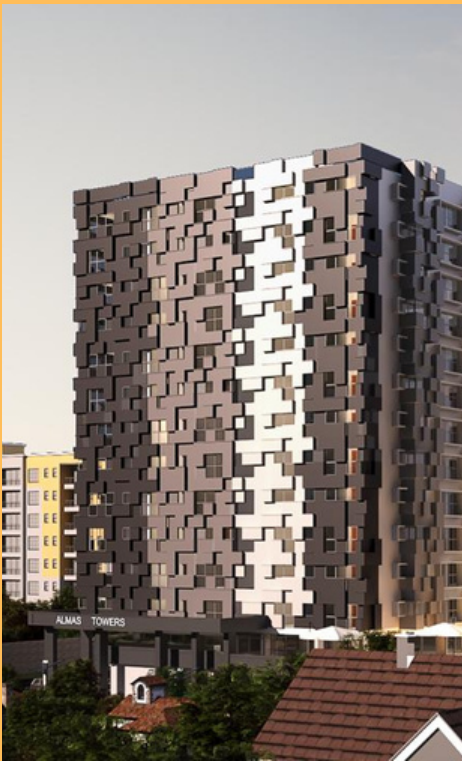
Almas Towers, 6 unit elevators.
