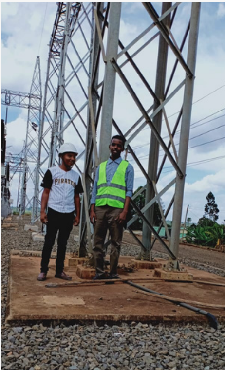
Linesman Ndiwa working on a 66 kv HT line at ndenderu Kiambu
