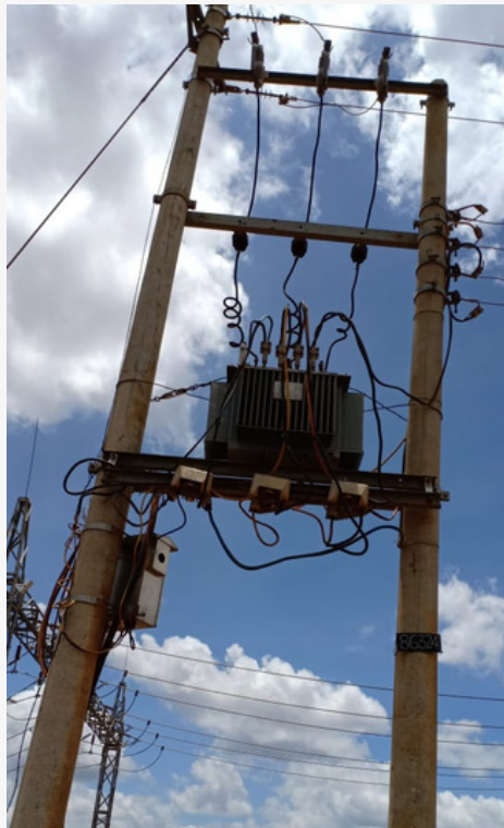
Preparation of 120 Kva mounting at Malaba
