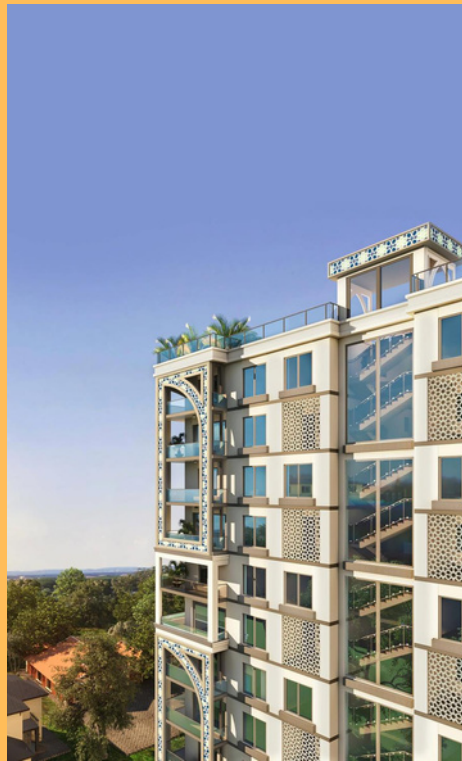
Tamam Residency, 6 unit elevators.
